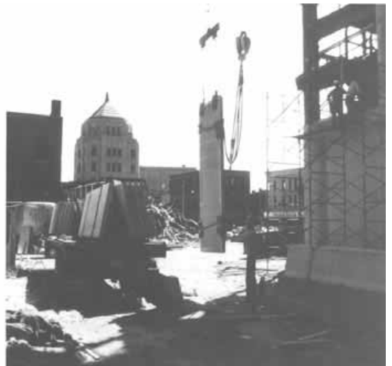
Turning a large panel in the air requires a crane with double mainfalls. This maneuver saves stacking space and reduces handling.
