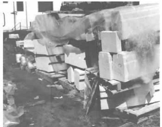
A messy, disorganized stacking yard like this will cost you money, time and trouble. Keep stone stacked neatly, and in setting sequence.
