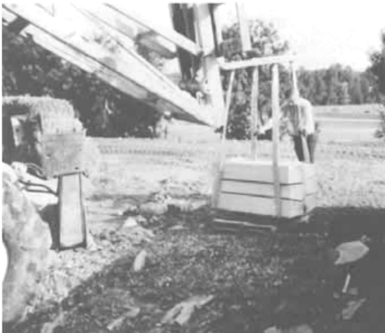
When unloading using slings, stack stones back to back, or insert padding between them to avoid chips from bumping.
