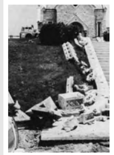
Before. Rails destroyed by a tornado.
