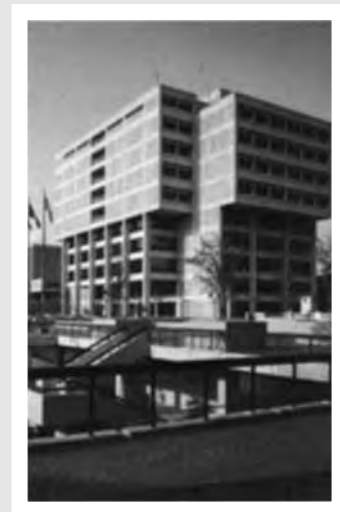
Civic Center Government Building, Baton Rouge, La.
