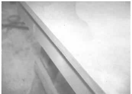
8 The completed repair will be nearly invisible.
