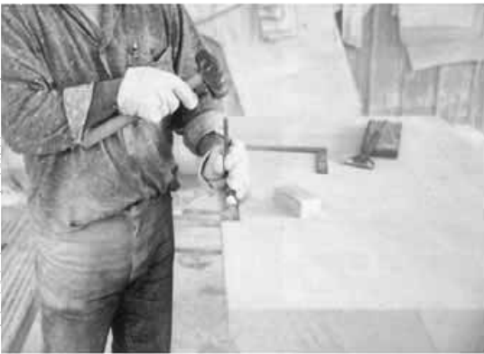
3 Square up the chipped area into a regular slot.
