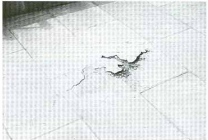
Over relatively few years, a snow-removal program using salt produced this deterioration on walkway paving.
